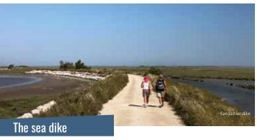
The sea dike ("digue à la mer") was built in 1859 to protect the Camarque from sea flooding. Water exchanged between the sea and the ponds now goes through sluice gates called "pertuis".
