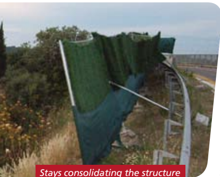
Stays consolidating the structure against the wind. © S. Fourasté
